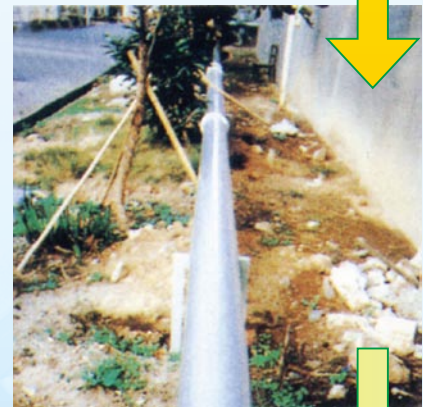
▲ 約40M水平輸送 Horizontal transport for about 40 meters.
