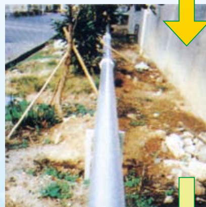
▲ 約40M水平輸送 Horizontal transport for about 40 meters.
